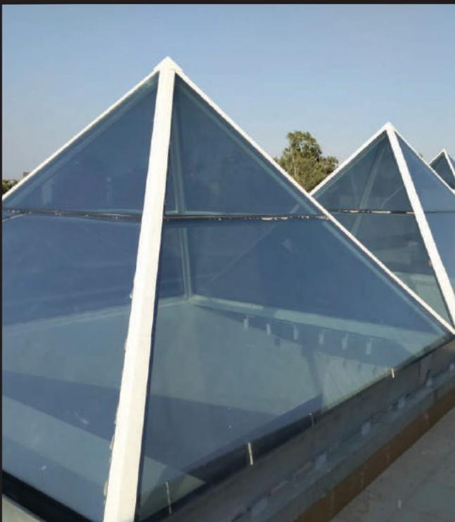
• **Final Result:** We have successfully installed three glass pyramid skylights with the required heat parameters and drainage system.
